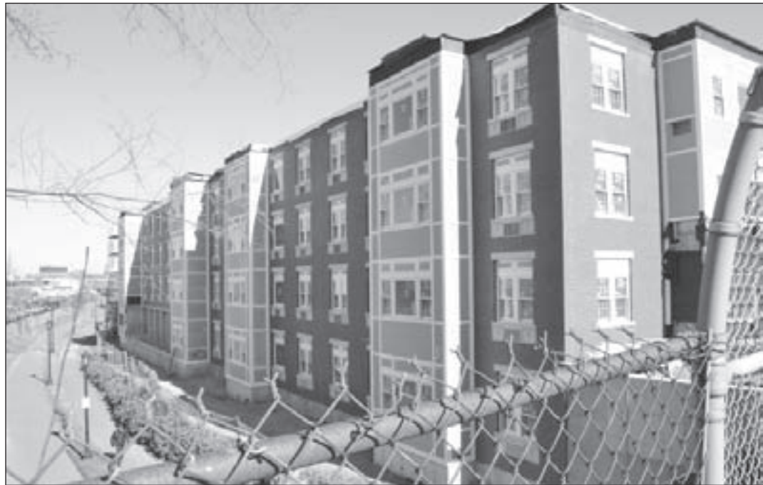
Construction on 27 new affordable apartments on Maverick Street for low-income families is well underway and should be completed this spring.
