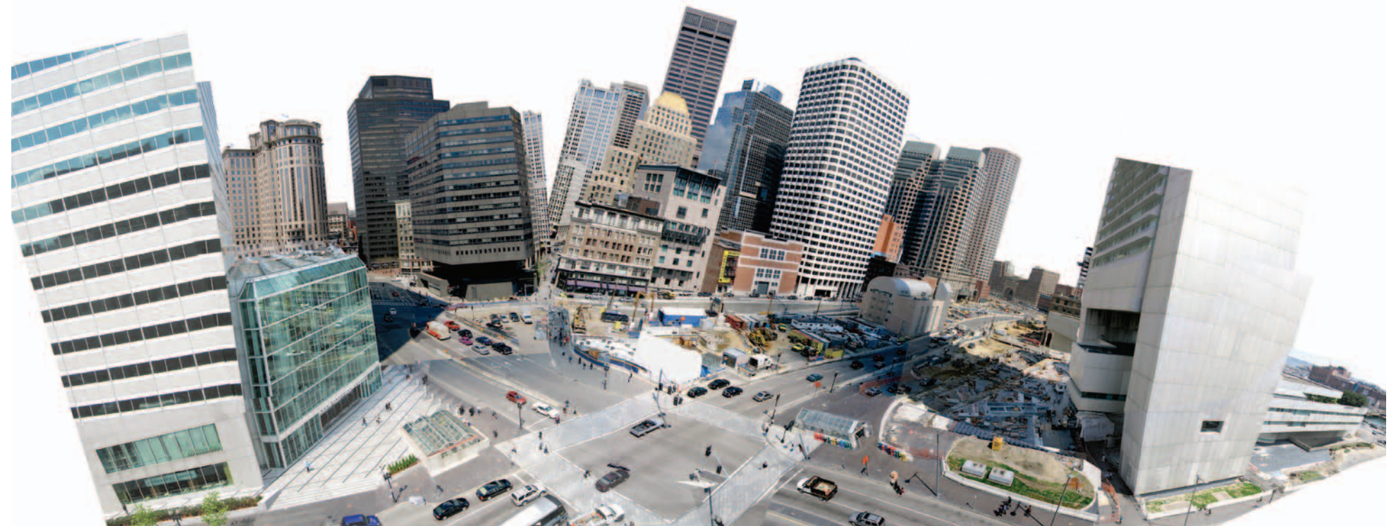
View of Dewey Square from South Station
